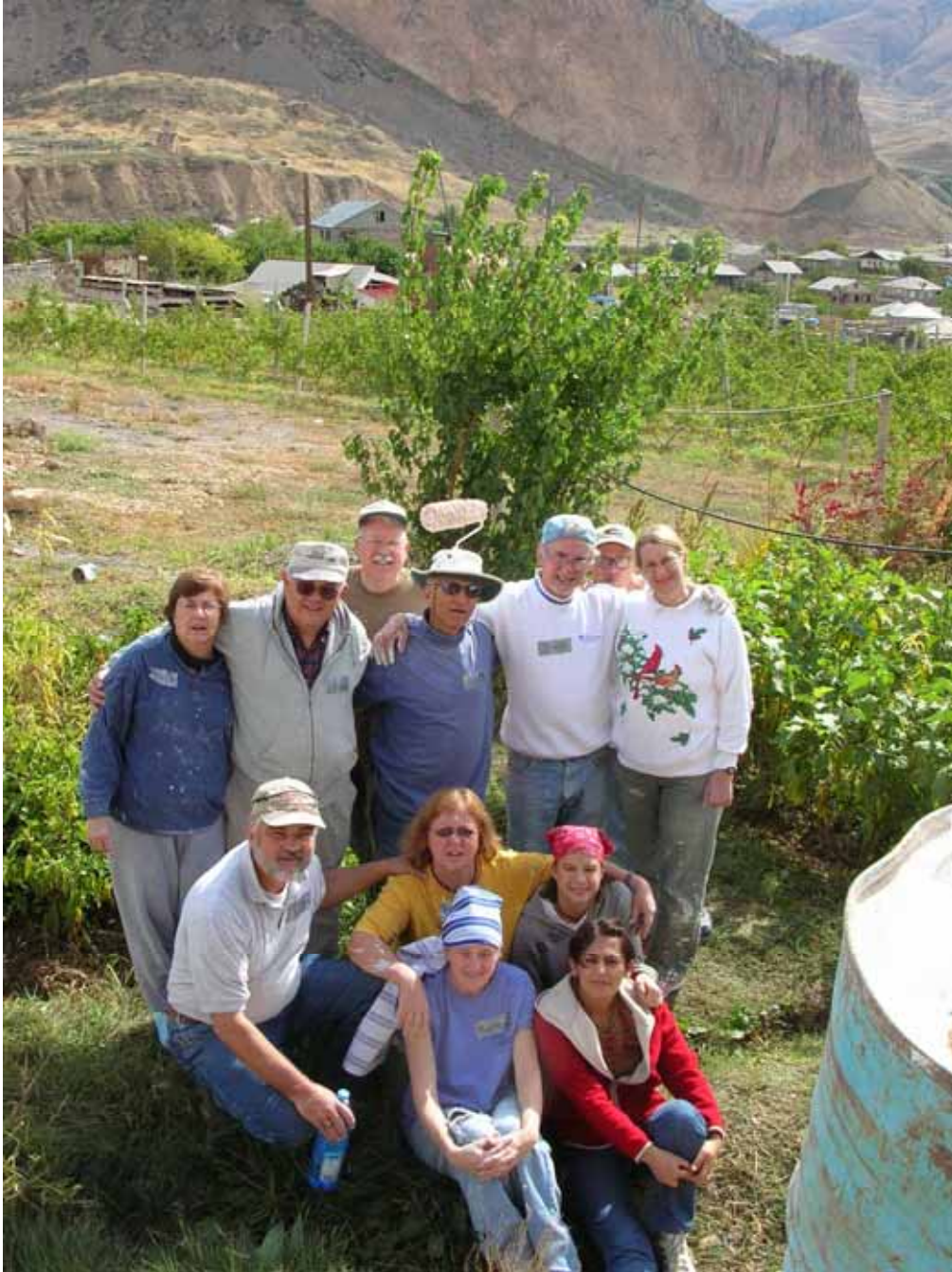
Pamela Karg (center) with members of the United Methodist Volunteers in Mission team from Ohio, as well as a Peace Corps volunteer and a Canadian-Armenian while working on a Habitat for Humanity house in the village of Areni (background). In addition to writing and editing grant proposals at the United Methodist Committee on Relief office in Armenia, Karg's volunteer duties include in-country coordination for volunteer teams which are open to anyone who has an interest in seeing the world through a different type of travel.
